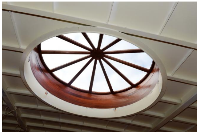
Figure 20 – Saloon ceiling showing round deckhouse.
