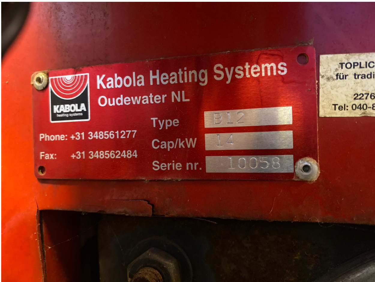
Figure 20 – Kabola Diesel Fired Boiler Nameplate
