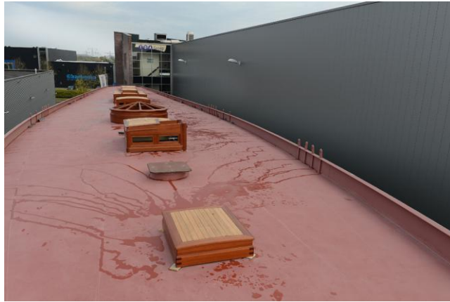
Figure 26 – Deck looking aft...
