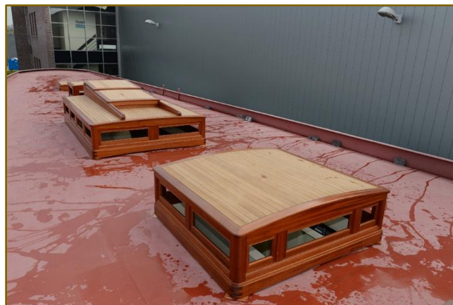
Figure 24 – Deckhouses from the bow looking aft.
